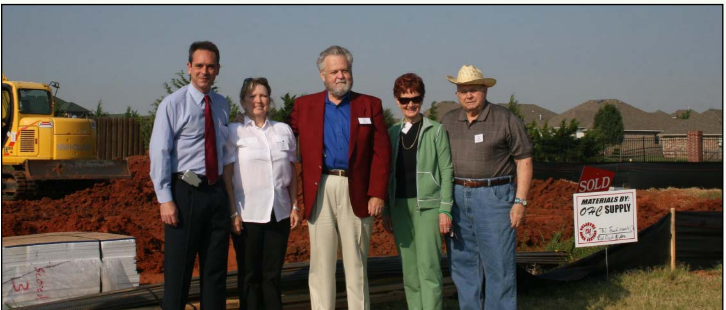
Touchmark at Coffee Creek Executive Director Jamie Ham, left, joins Margaret Neville and Richard Neville as ground is broken on their Parkview home recently. With them are Liz and Bob Kelly, right, who also are getting ready to build their house next door to the Newvilles.
